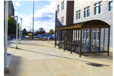
Transit (Barrel Roof)
